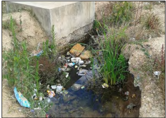
Clean water from a burst water pipe, now polluted. Masvingo. Photo by Entrance Takaidza, HCC photographer,
